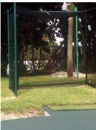
Renovated chipping net
