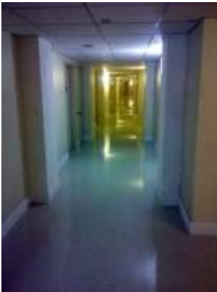
New north tower 1st floor hallway
