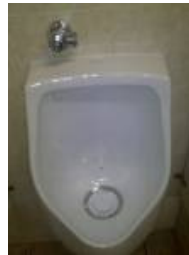
New waterless urinal -- Picture included for those women who have not recently toured the men's rooms in the common spaces
